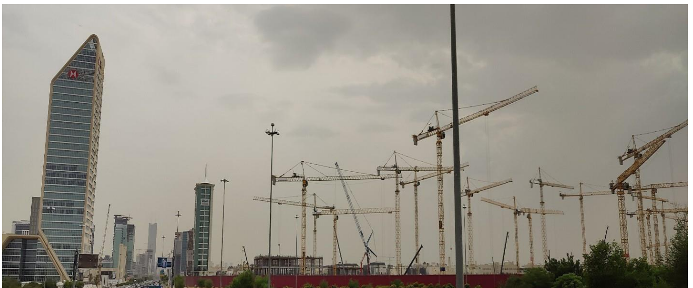
Riyadh under construction.
